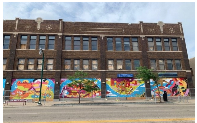
Coliseum Building on Lake Street & 27th Avenue Authentic Restoration Photo
